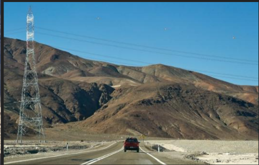
Paved highway & 2 powerlines cross the property (550 & 22KV)
