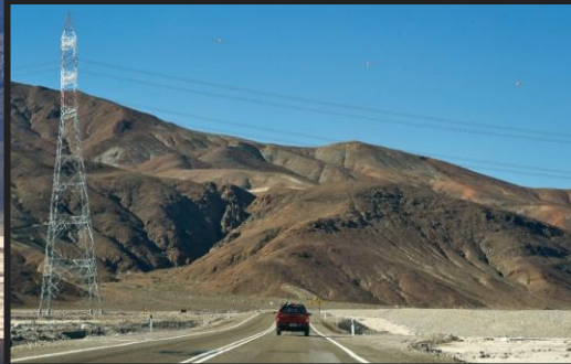
Paved highway & 2 powerlines cross the property (550 & 22KV)
