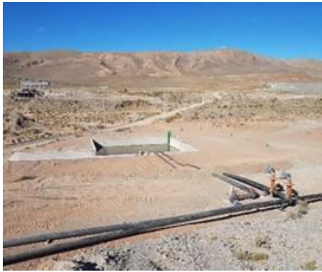
Tailings Pumps Emergency Pond
