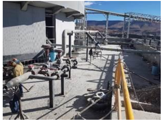
Tailing – Dilution System
